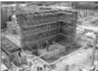
Unit 1 Transformer Foundation
