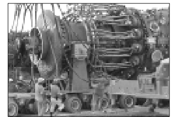
Turbine Unit 1 Installation
