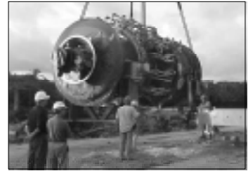
Turbine Unit 1 Installation
